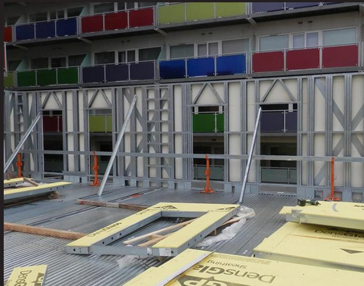
Maximising state-of-the-art digital and offsite technology the specialist team at Frameclad designed engineered and manufactured an advanced loadbearing steel frame solution (SFS) using a full Building Information Modelling (BIM) approach with customised Tekla software. Using Frameclad's loadbearing frames provided multiple benefits to the project, including faster and safer installation to help speed up the building programme.
