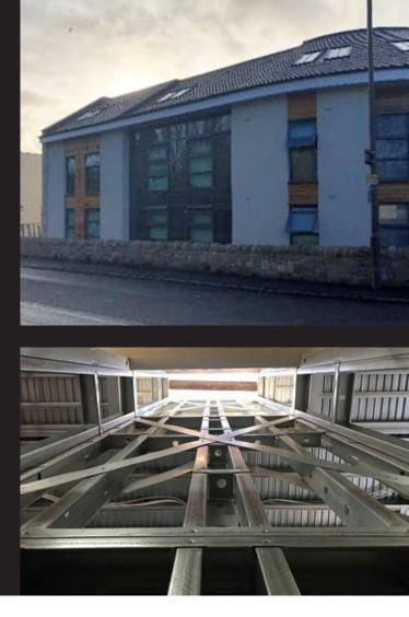
Frameclad worked with the main contractor and client to meet the specific needs of the project, which stipulated the use of some of the previous building's original stonework. This was incorporated into the external cladding of the building. The cottage-style building offered a complex challenge, which required several SFS frames and techniques to achieve the desired result.
